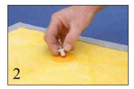
Insert marking plugs into the Snap-On anchors.
