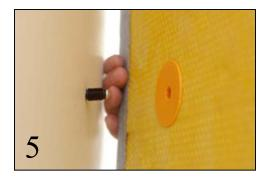
Firmly push panel onto ratchets to complete installation.
