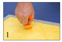
Screw Snap-On Anchors into the back of the panel using the driver tool.
